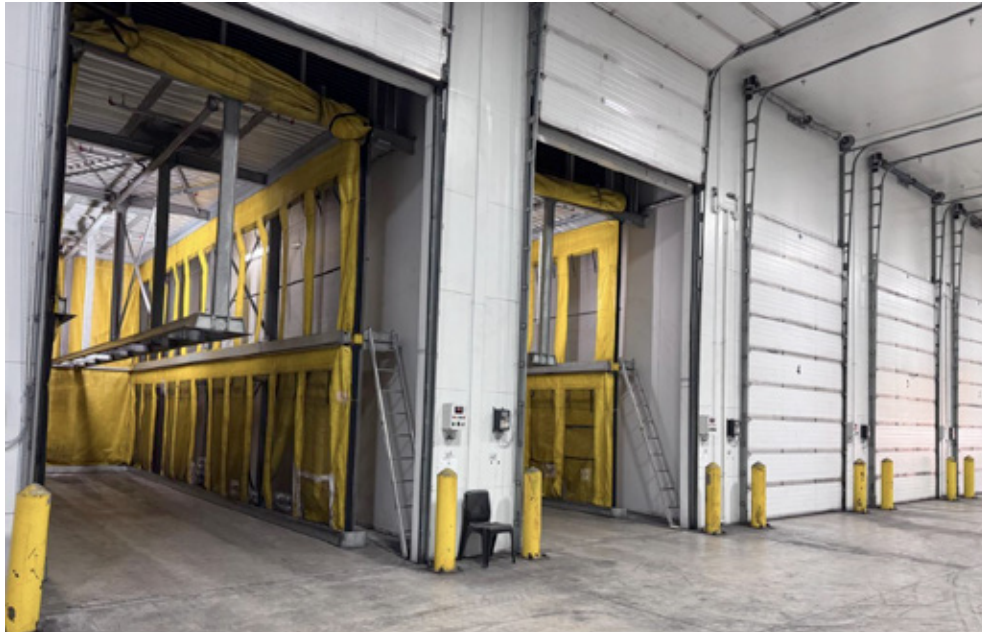
Cold treatment chambers
